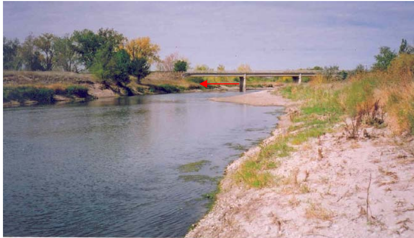
Figure 4.3b. Looking upstream toward the Keystone bridge. Note the incised geometry of banks and break in bank line consistent with top of form line on piers.
