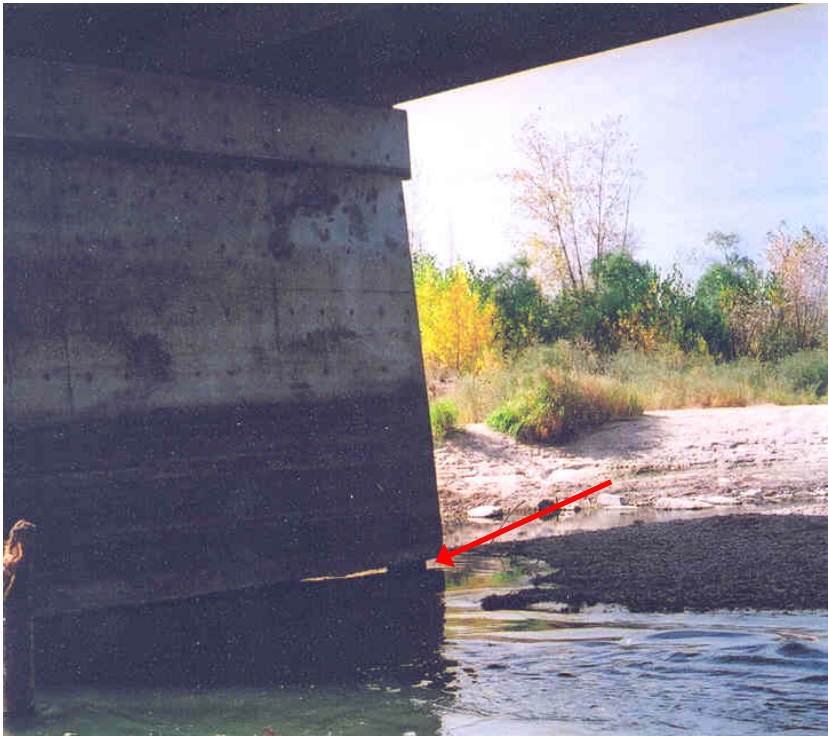
Figure 4.3d. Looking at the upstream end of the Keystone bridge pier, showing the gap between the base of the pier and the water surface. The outline of the exposed foundation pile is discernable in the gap.
