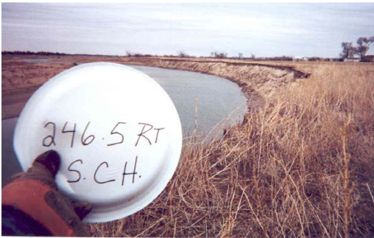
Figure 4.4b left. Looking downstream along the south channel, immediately downstream of J2 return (RM 246.5). The channel is deeply incised with steep high banks.
